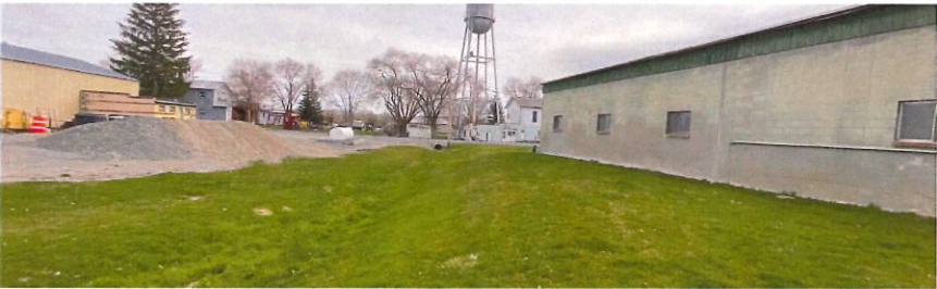
DRAINAGE DITCH AT BACK OF BUILDING
