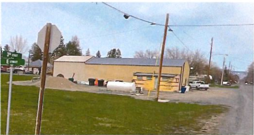
EXISTING BUILDING AT NORTH LOT
